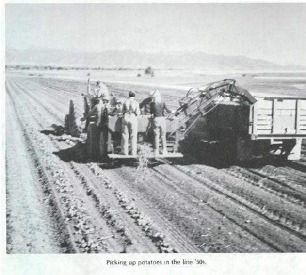
Picking up potatoes in the late 50s. Potato combine built by Wilbur in the early 1950s.
