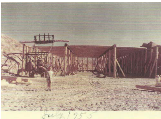
John & Rudy Broksle built this cellar in 1958. The roof is laid with twigs, straw bales, dirt and then tin. The concrete floor was added in the 1970s. The structure is still in limited use today. Sherrie Broksle is in the foreground riding her stick horse.
