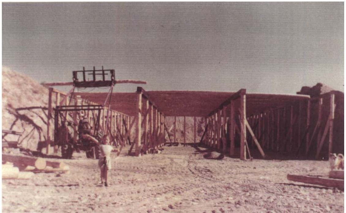
Erection of a storage building on the John and Rudy Broksle's farm in 1955.
