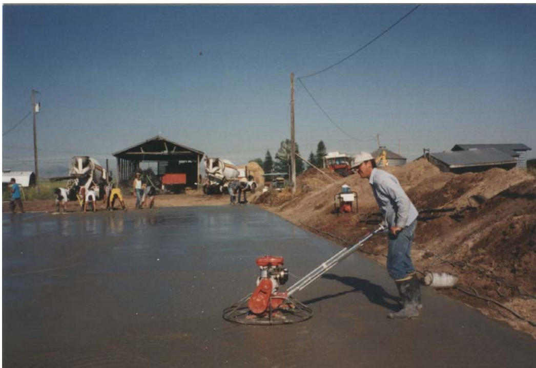
Pouring concrete for the Lake Brother's storage facility near Ronan in 1994.
